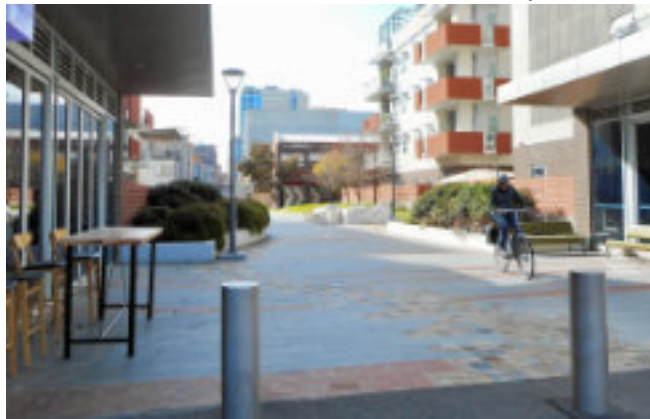
Minor Works Building on Sturt Street East ... not easily found behind the Ergo Apartment buildings
